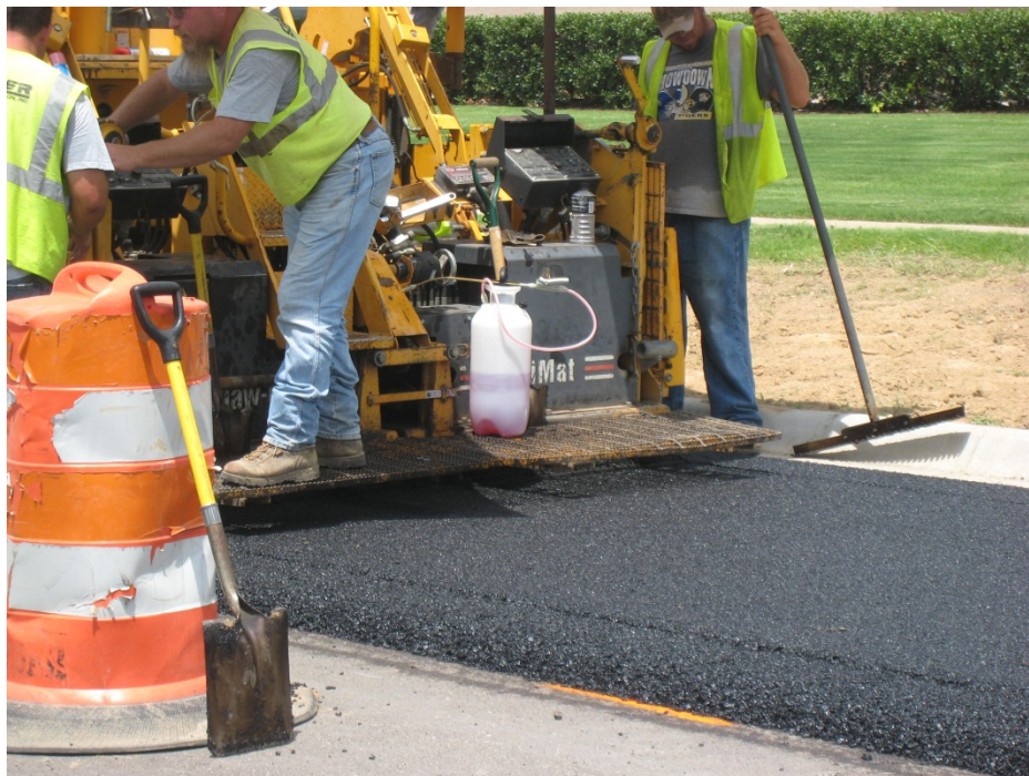
Figure 89. Fayetteville Warm Mix Section Under Construction
