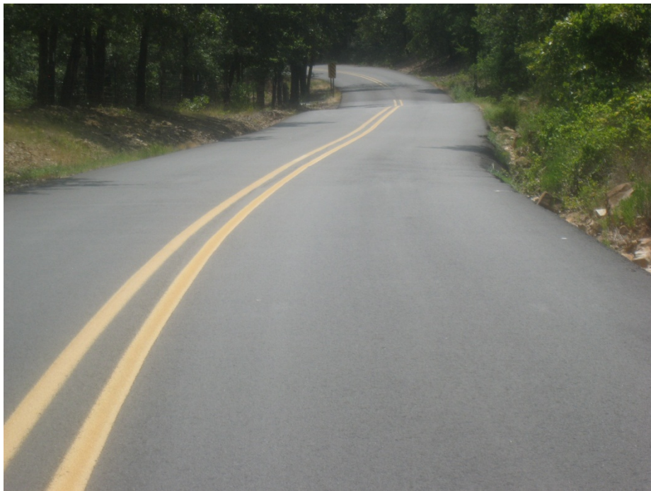
Figure 87. Faulkner County Warm Mix Section After 3 Years in Service
