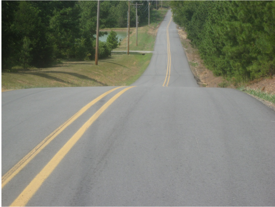
Figure 88. Faulkner County Hot Mix Section After 3 Years in Service
